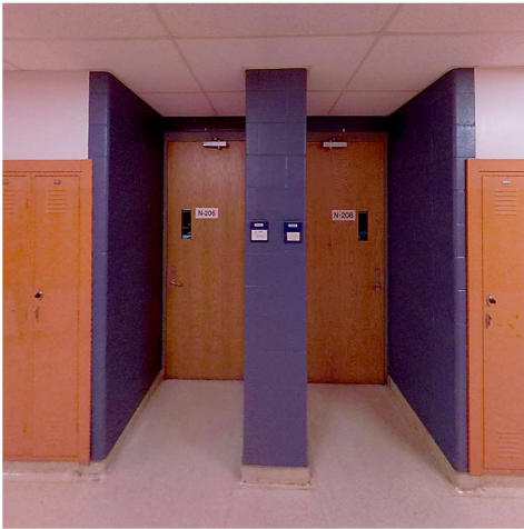
AAB Non-Compliance: Doors lack pull side clearance, typical for numerous doors
