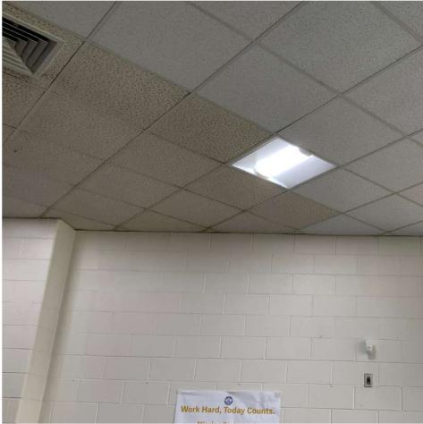
All ACT ceilings are extensively damaged, cracked, stained and mismatched
