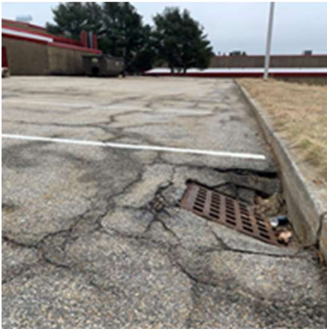
Vehicular and pedestrian pavement and curbing is in poor condition throughout the site
