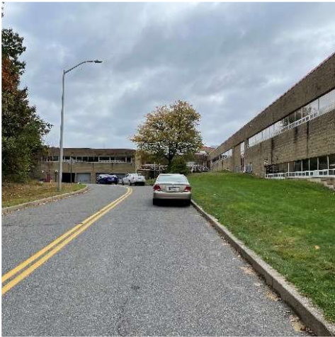
Poor exterior envelope performance
